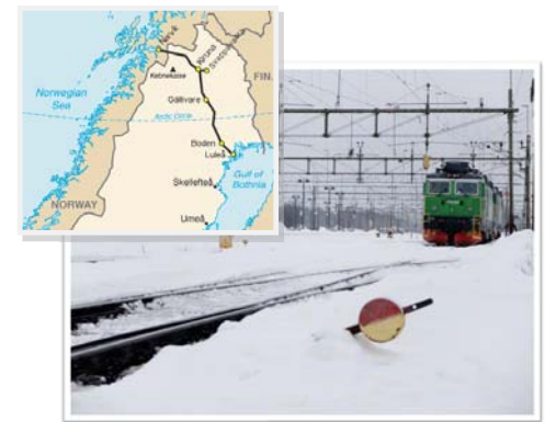
Railway corridor , Iron Ore Line in Malmbannan in northern Sweden, managed by Trafikverket
